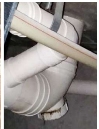
Figure 14: Worn rubber gasket
