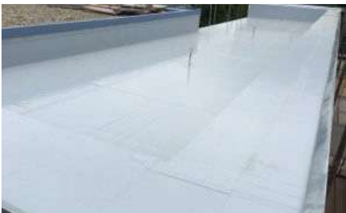
Figure 21: Permanently elastic and reflective Ketone Ethylene Ester Single Ply Membranes
