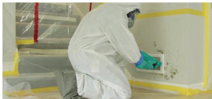
Figure 4: Personal Protective Equipment during Mold Remediation Cleaning
