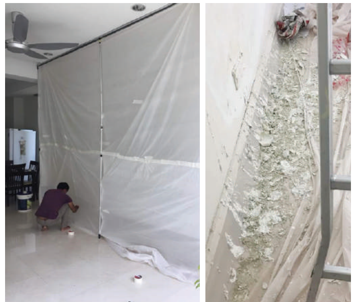
Figure 5: Mold remediation with physical removal of mold
