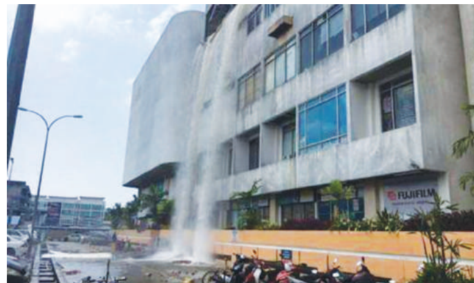
Figure 1: Burst water tank in a 4-storey shopping mall in Kuantan in 2017
